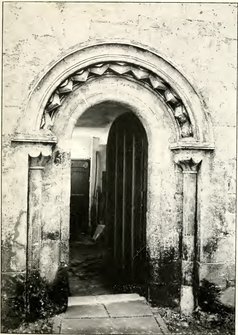
FIG. 3.—HORTON MANOR HOUSE, NORTH DOORWAY.
